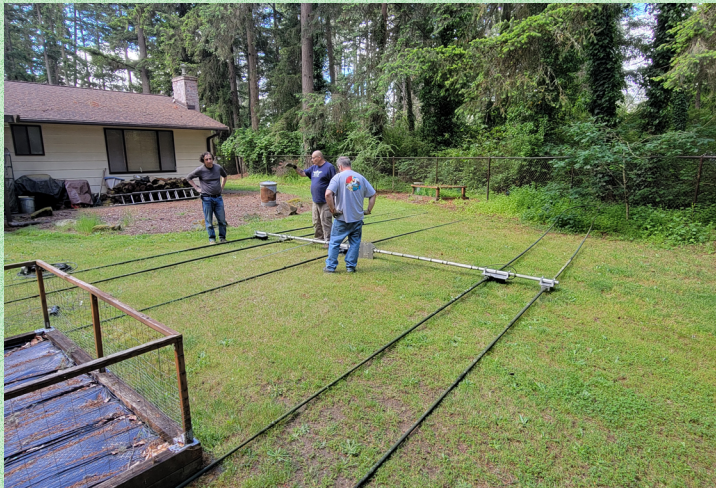
Successful removal of DB-18 from the tower. Large footprint! Now ready for disassembly.
