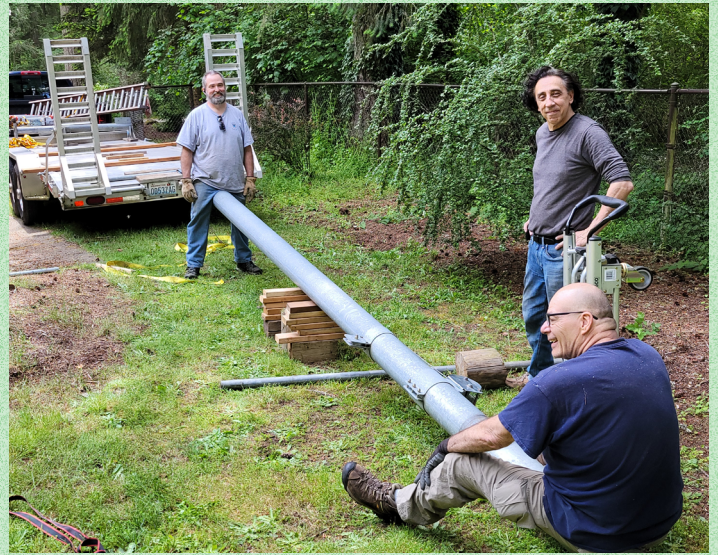
Employing teeter-totter technology to gain elevation to load the tower.
