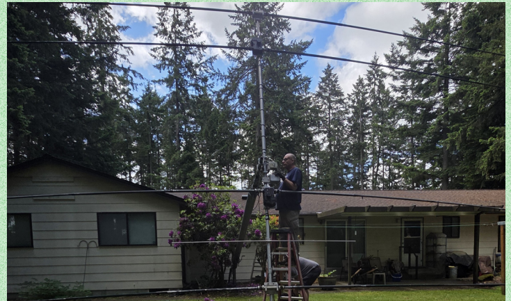
BJ KO7T removing DB-18 from the tower.
